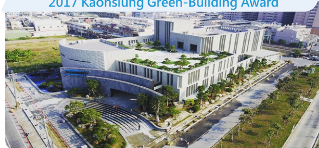
Cleanaway Group: 2017 Kaohsiung Green-Building Award
